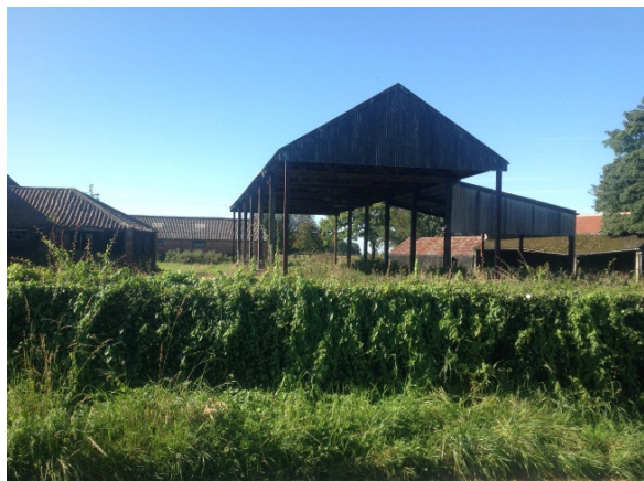
Fig 33: Village Farm sheds and Outbuildings
