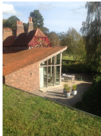
Fig 11: Oak roof at the Horse Engine House, Village Farm Fig 12: Modern extension at Midsummer Cottage uses local handmade brick and incorporates a structural oak frame
