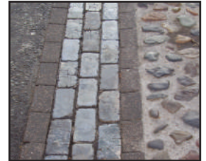
Granite sett drainage channels
