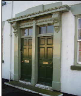
Six panel doors with glazed fanlights
