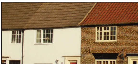
Windows set close below the eaves
