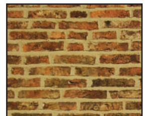
Modern cement pointing
