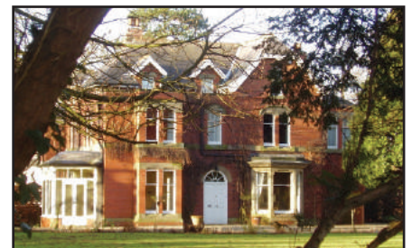
Leven Bridge House/Levenside House - Late 18th Century
