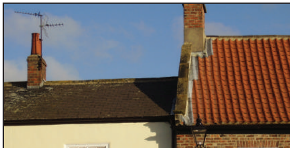
Slate and pantile roof coverings
