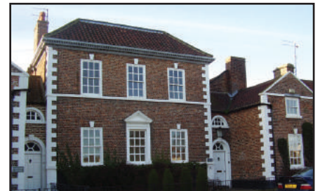
Handyside House - Mid 18th Century
