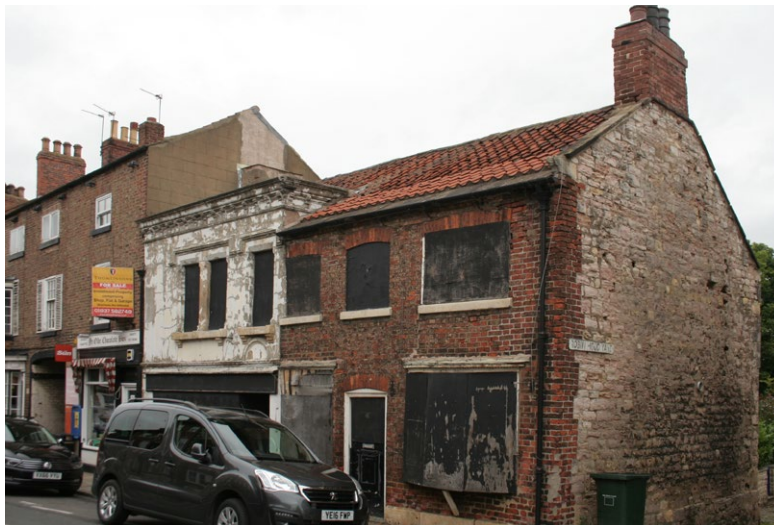
Brick facing on an earlier limestone construction at 24 Kirkgate. Note the dilapidation on this and the neighbouring building
