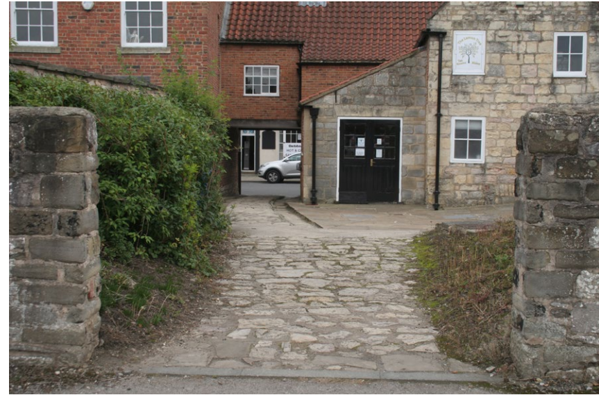
View of a side passage from High Street to the central car park with traditional and original York stone setts and York stone slabs that are probably not original
