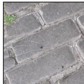
Timber pavers, Johnson's Yard
