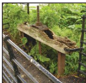
Sluice gate
