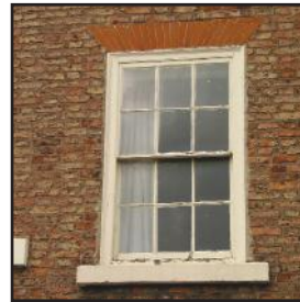
Rubbed brick window heads
