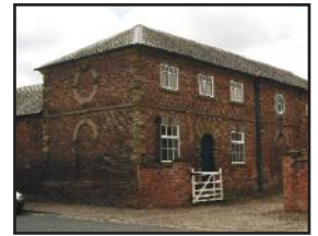
Stable buildings, Thirsk Hall
