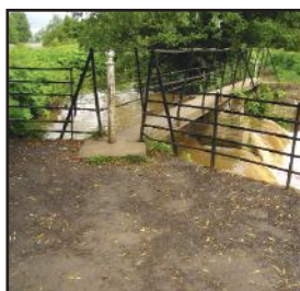
Wrought iron fencing at Cod Beck
