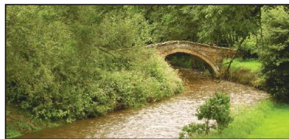
Town End Bridge
