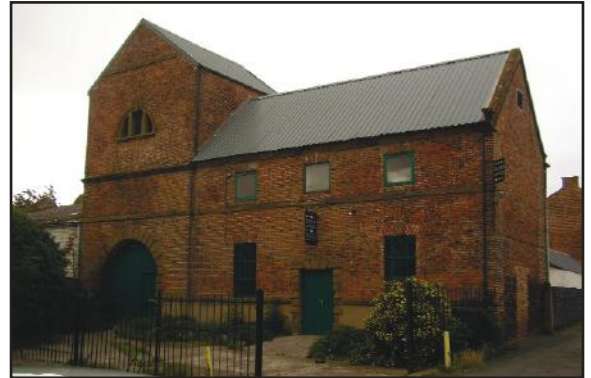
Old Stable Block, Chapel Street
