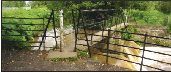
Sluice gate, The Holmes
