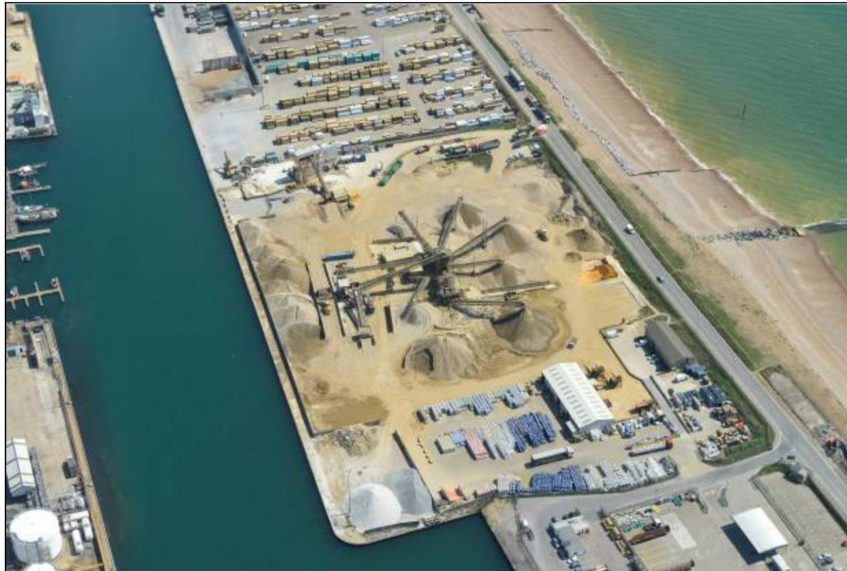
Photograph 8: Tarmac Marine Dredging's large scale aggregate wharf Shoreham East Port (courtesy of Hanson UK).
