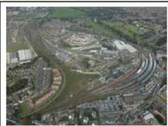
York Central. The largest brownfield site in Europe next to a railway station
