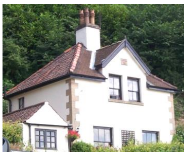
Crag Cottage, Main Street: central chimney stack
