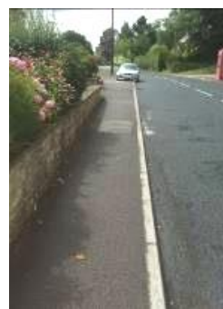
Concrete kerbing and tarmac footpaths erode rural character
