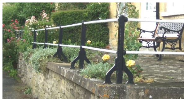
Cast iron railings along The Terrace
