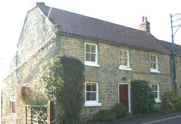
Abbey House, Main Street: coursed rubble to gable, squared stone to front
