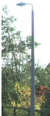
Concrete street light in Manor Close
