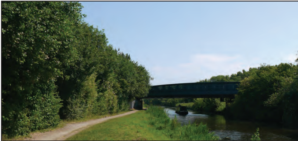
View along the Selby Canal to the railway bridge
