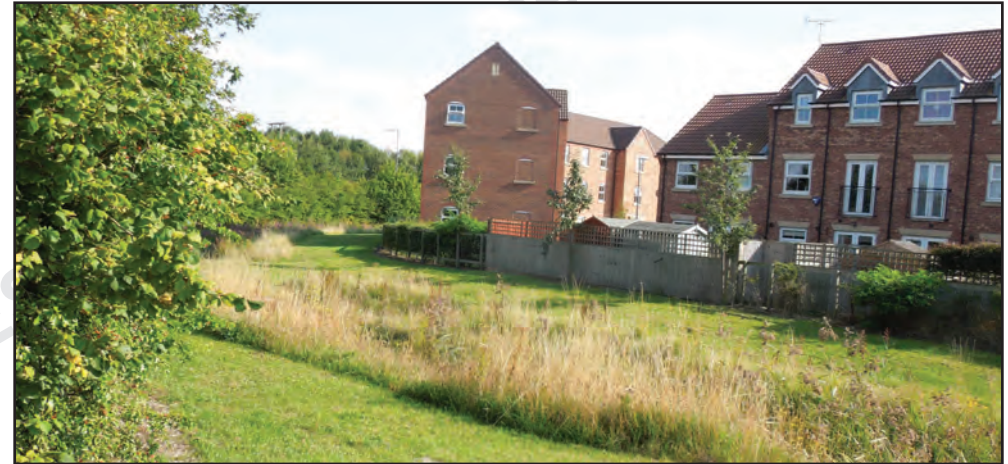
View of settlement boundary, drain and buffer planting along A63
