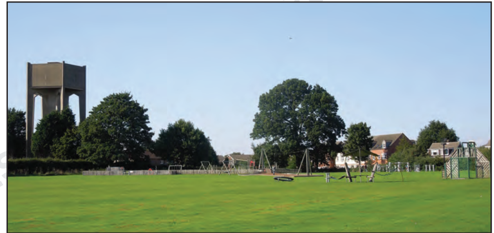
Play area to settlement edge with water tower
