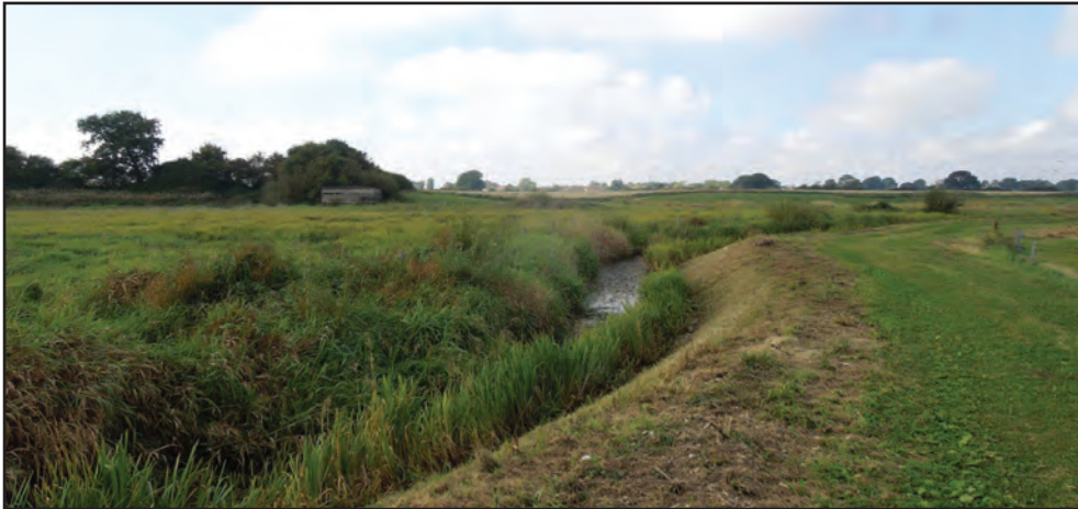
View from edge of washland area looking to village
