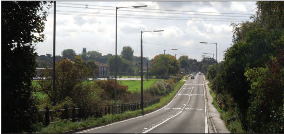
View down Station Road A1041 towards Carlton from railway bridge
