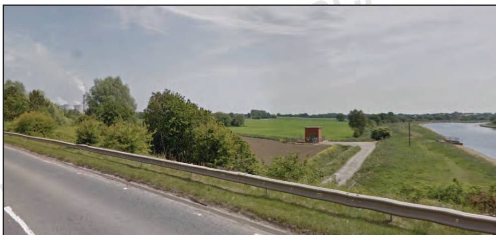
View north eastwards from A19 over Aire & Calder Navigation
