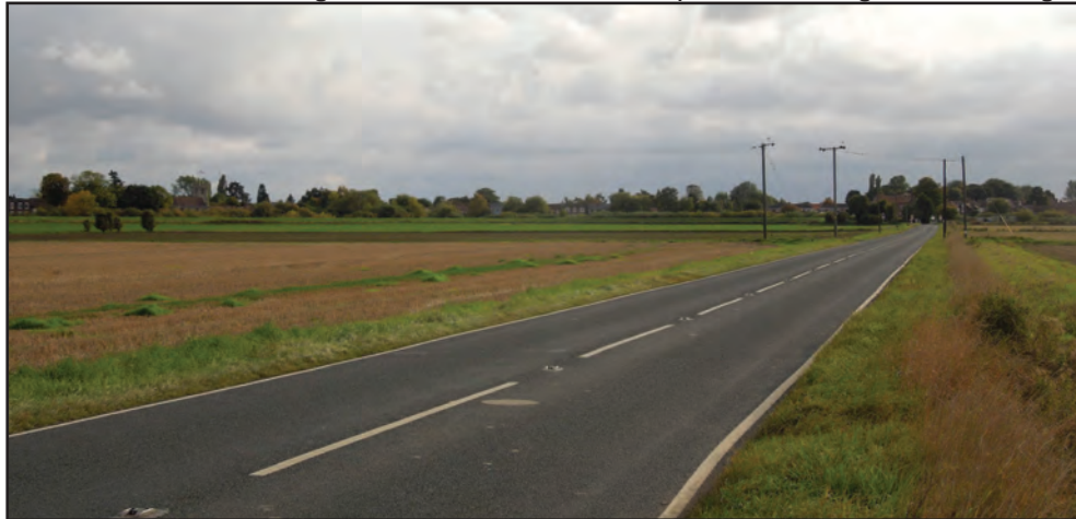
View from Kelfield Ings towards north side of Cawood
