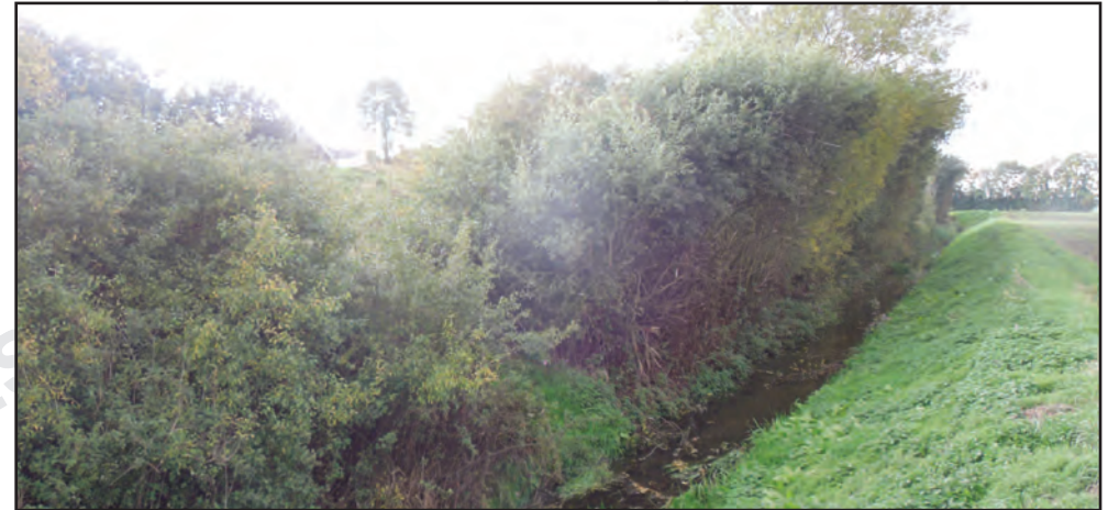
View west along dyke and flood defence bund north side of Kellington
