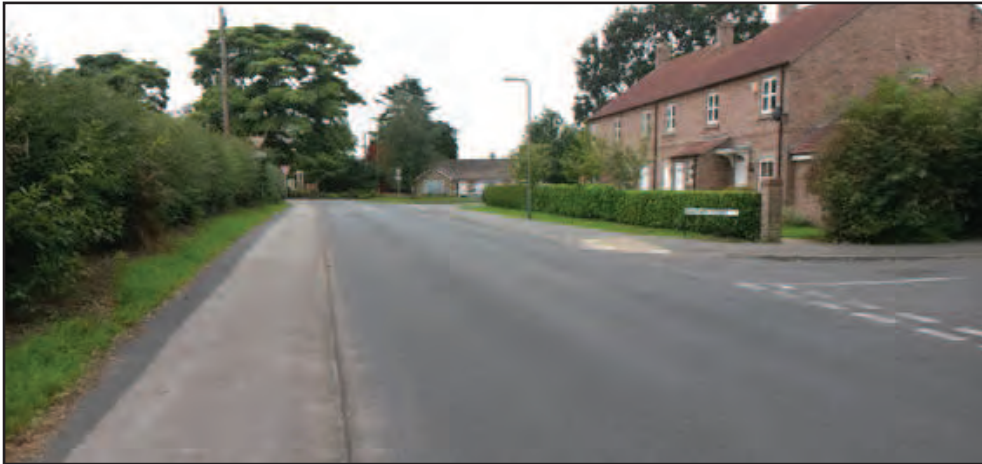
View south along the Baffam Lane
