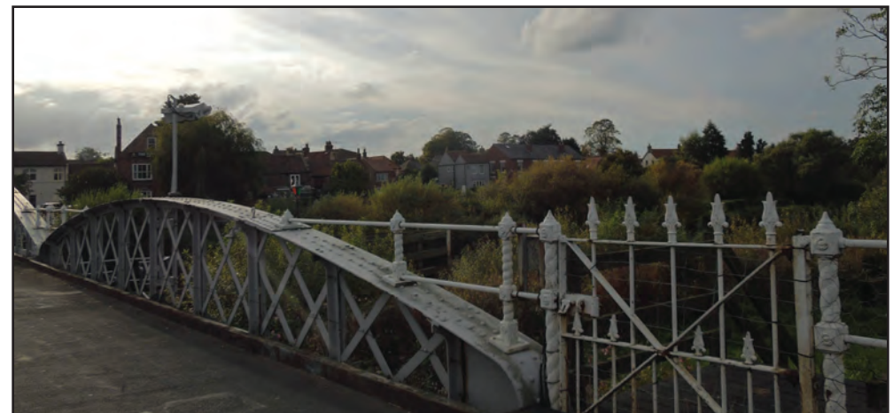
View to Cawood from swing bridge on B1222
