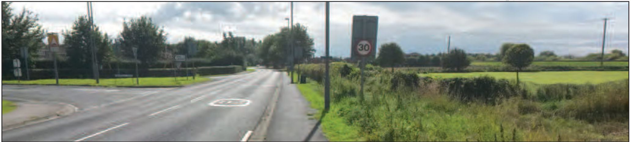
View south along Barlby Road
