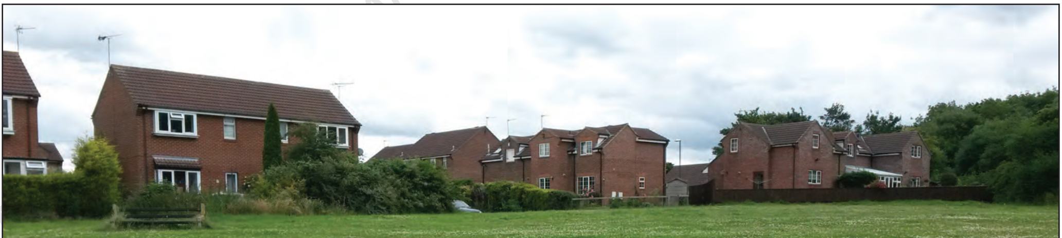
View of settlement edge at Kelcbar Close and Kelcbar Way
