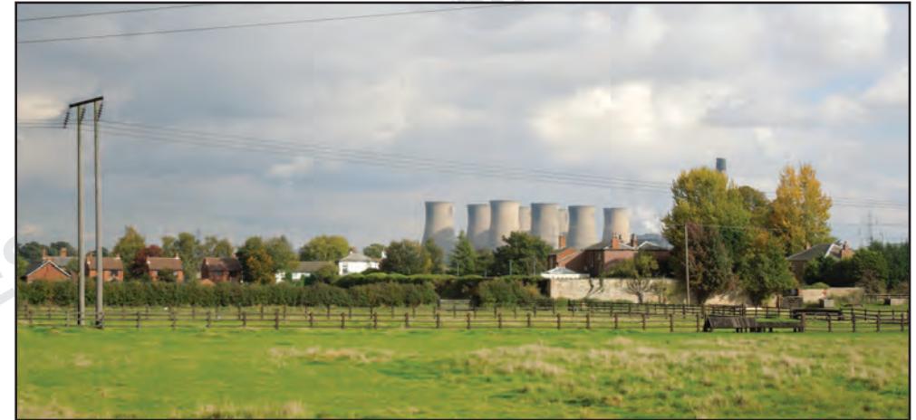
View east from Church Lane near St Edmunds Church
