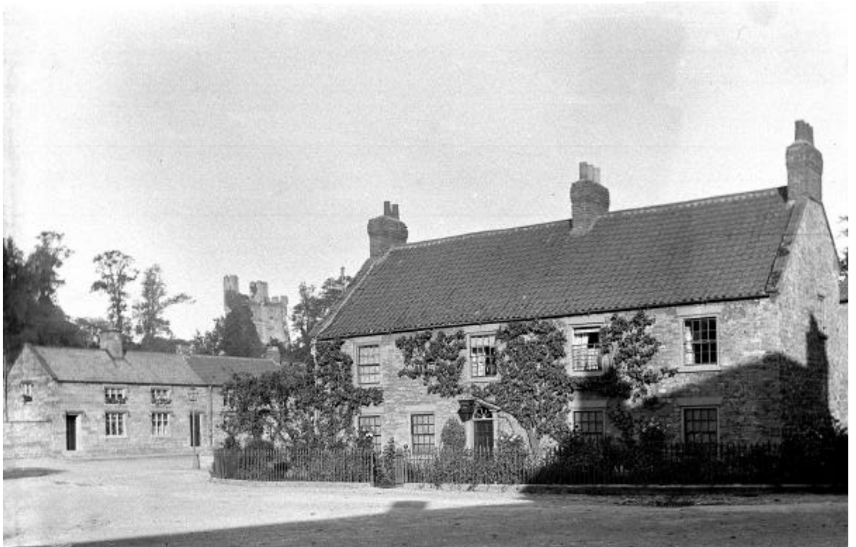
View of Buckingham Square from Bridge Street
