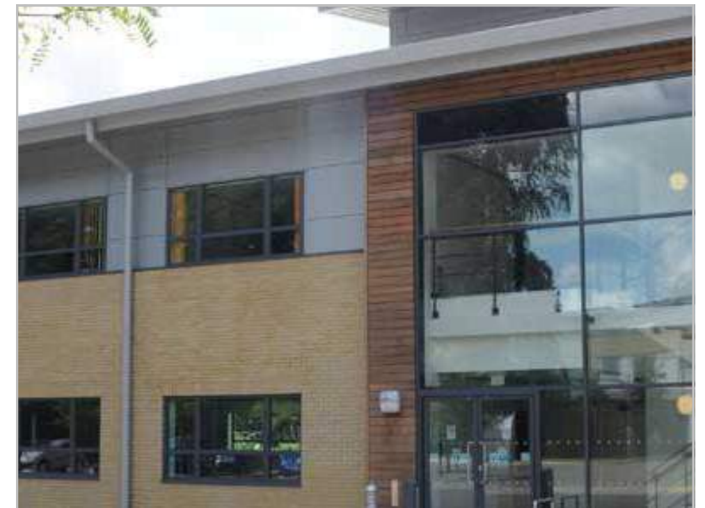
Good quality cladding panels raise the standard above the normal industrial park
