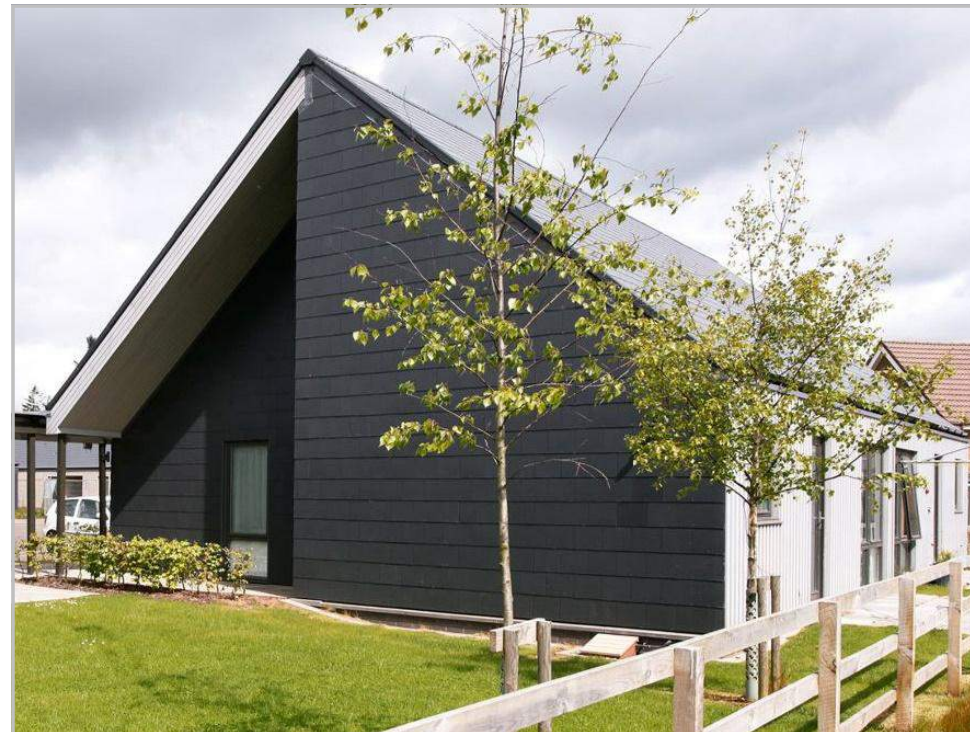
Artificial slate roofing and cladding fits a modern building into its context
