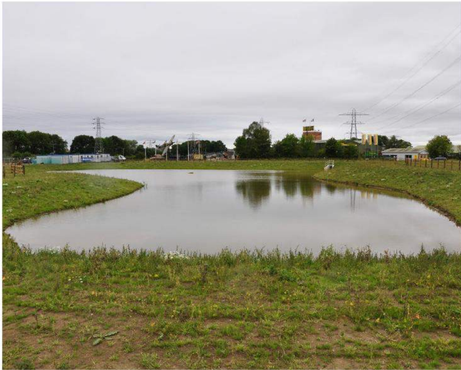
Photograph of completed retention pond in the southern field opposite Eden Camp.
