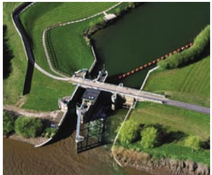
River Derwent and River Ouse at Barmby Barrage
