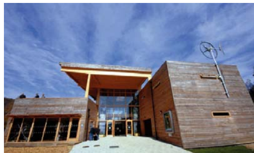
Figure 38 Building mounted wind turbine at Dalby Visitor centre in Ryedale (Source: Green design at Dalby visitor centre case study, Forestry Commission, 2010)
