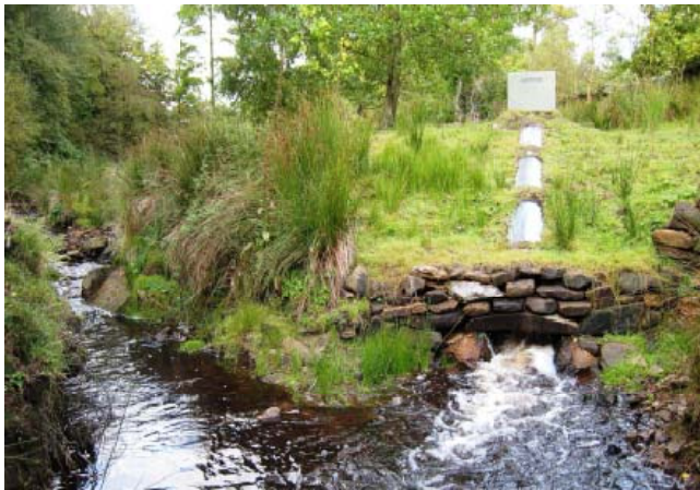
Figure 24 Bonfield Ghyll hydro facility in the North York Moors National Park (Source: Case study, Mann Power Consulting Ltd)
