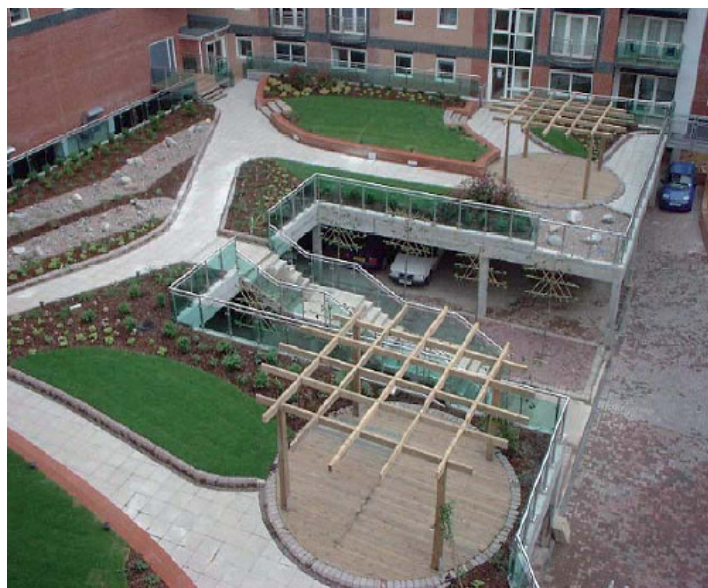
Figure 8-2: The Royal Plaza, Sheffield – Example of a Green Roof used within Residential Accommodation.
