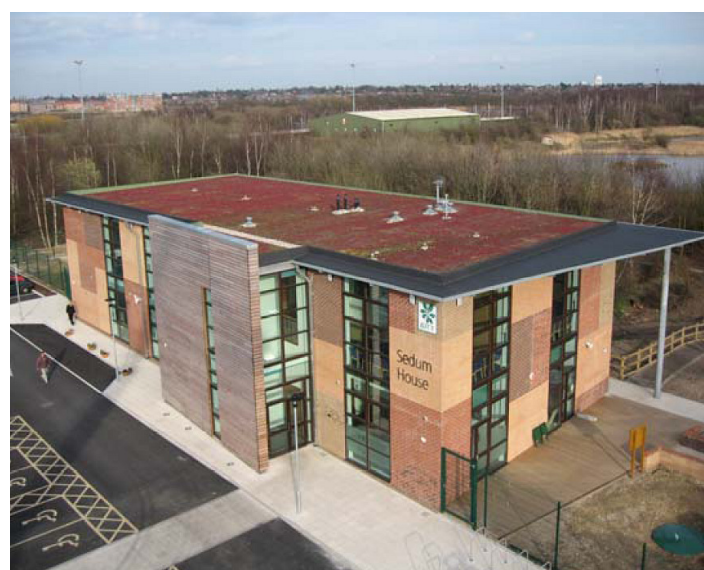
Figure 8-3: Sedum House, Doncaster – Example of a Sedum Roof used within a Commercial Development.
