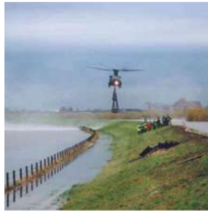
Selby's flood defences in the 2000 flood
