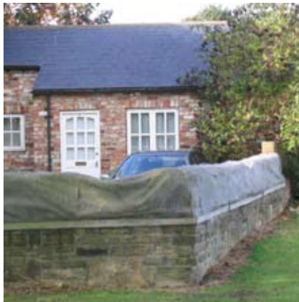
Temporary flood defences in Selby
