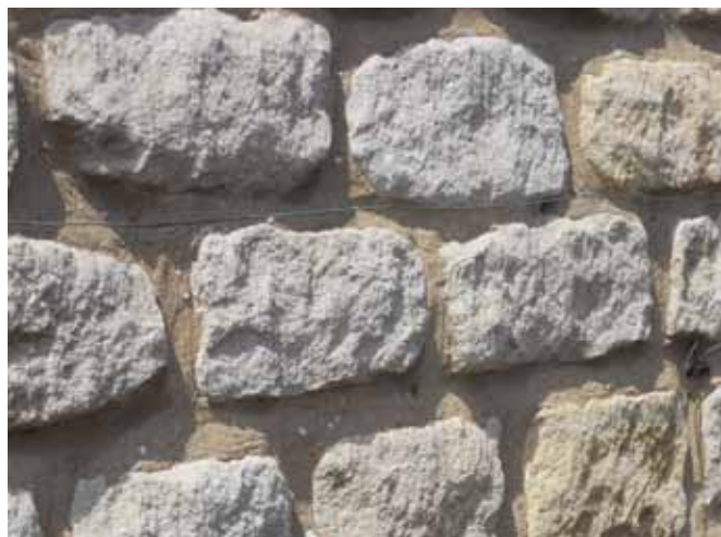
Recessed Bagged Pointing
