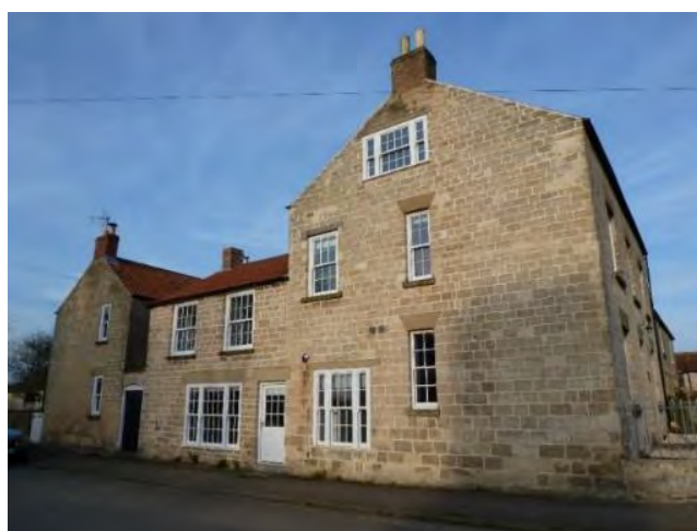
Lime pointing at Prospect House
