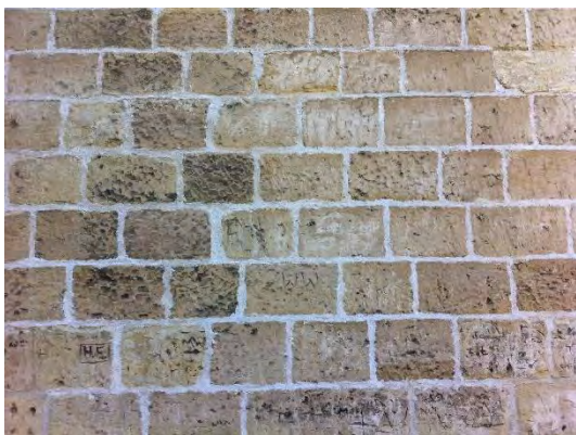
Lime mortar pointing
