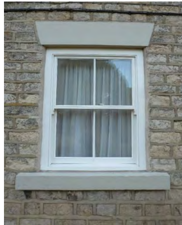
Modern sash window
