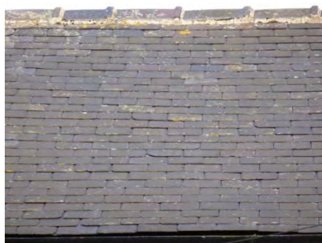
Natural slate roof
