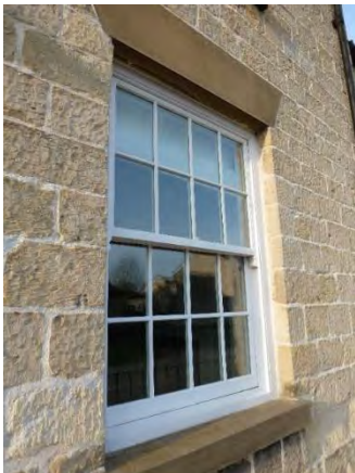
Modern sash window
