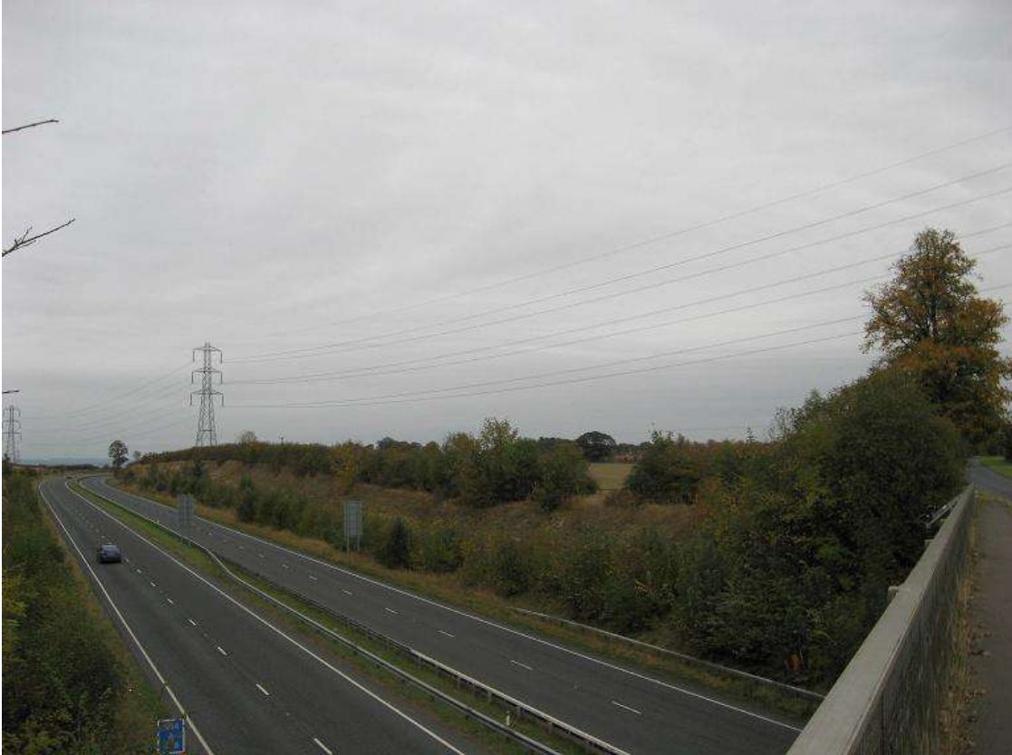
Figure 69 Castle Howard Road Bridge looking north SE 771(E) 714(N)
