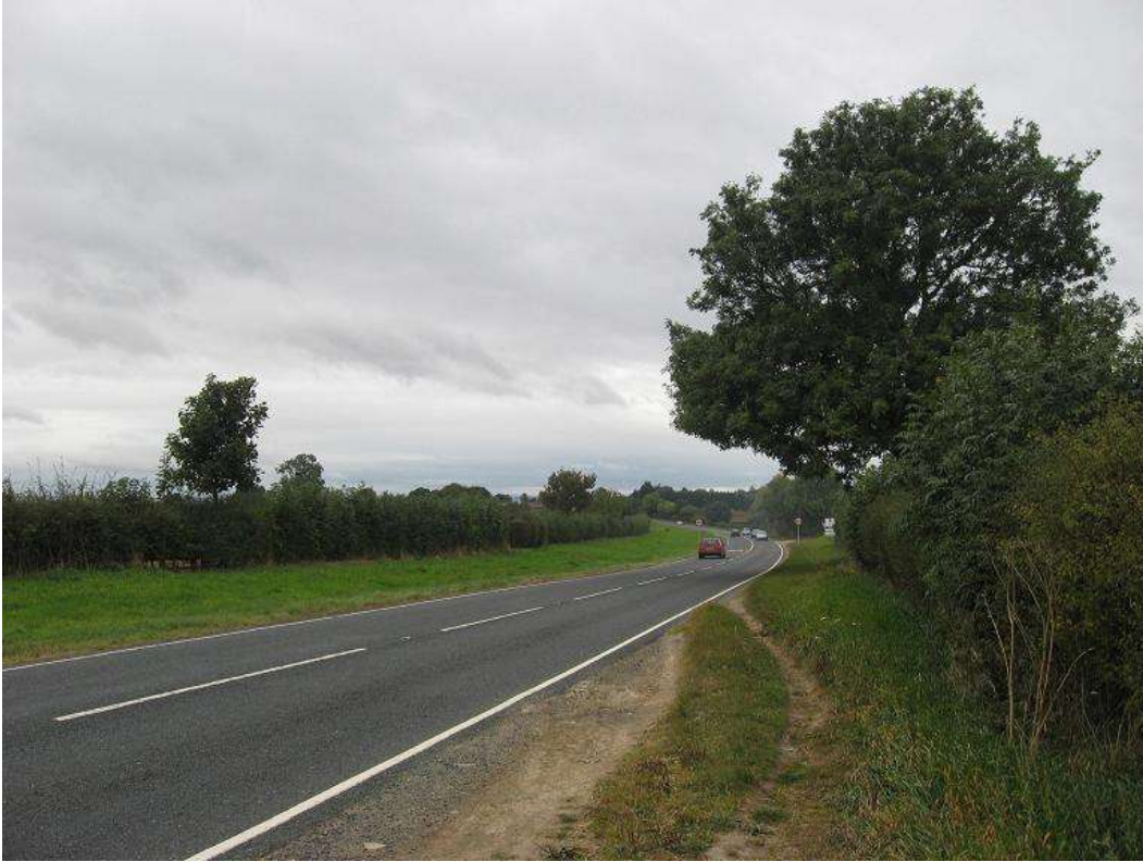
Figure 86 A169 looking southwest, broad location PH4 is where the road bends to the left SE 808(E) 847(N)
