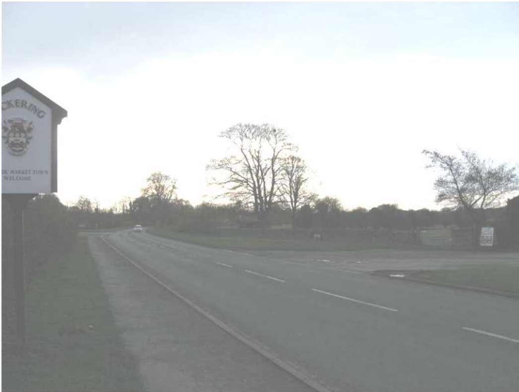
Figure 85 A170, edge of Middleton, looking south-east, towards Keld Head SE 785 (E) 850 (N)
