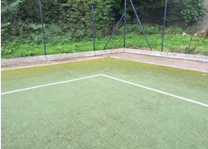
Figure 1.2: The image below illustrates the lines of the pitch lifting, creating a trip hazard.
