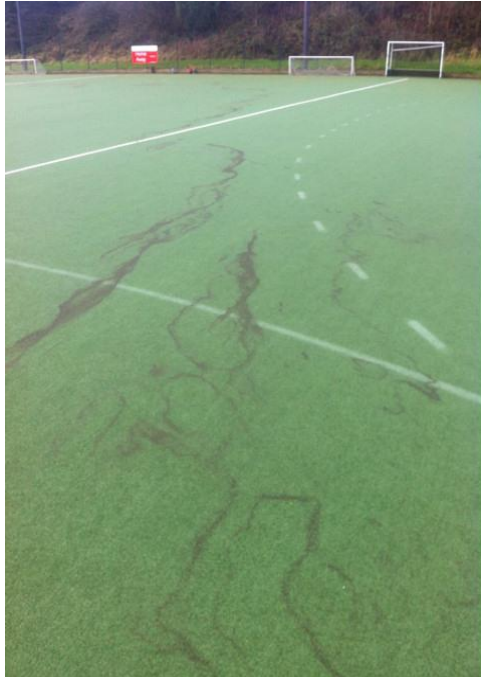
Figure 1.1: The image below illustrates the short pile and moss infestation at the surface of the AGP.
